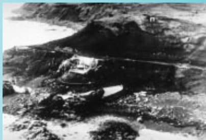
Scotch Cap Lighthouse after tsunami
